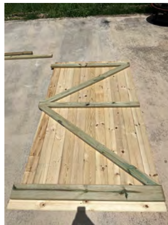
Figure 13 Purchase and construction process of the door made from new lumber
