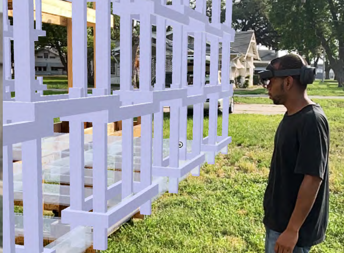
Figure 88 The overlay of the digital model with the assembled blocks
