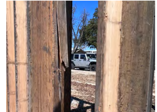
Figure 62 Defect in the framing stud
