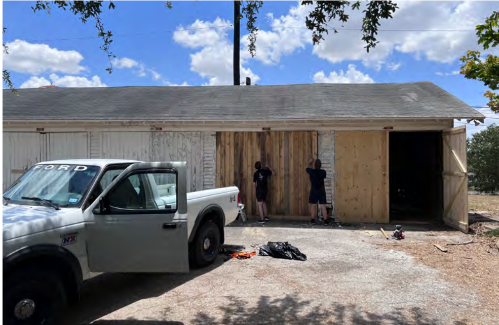
Figure 19 Installation of the reclaimed door
