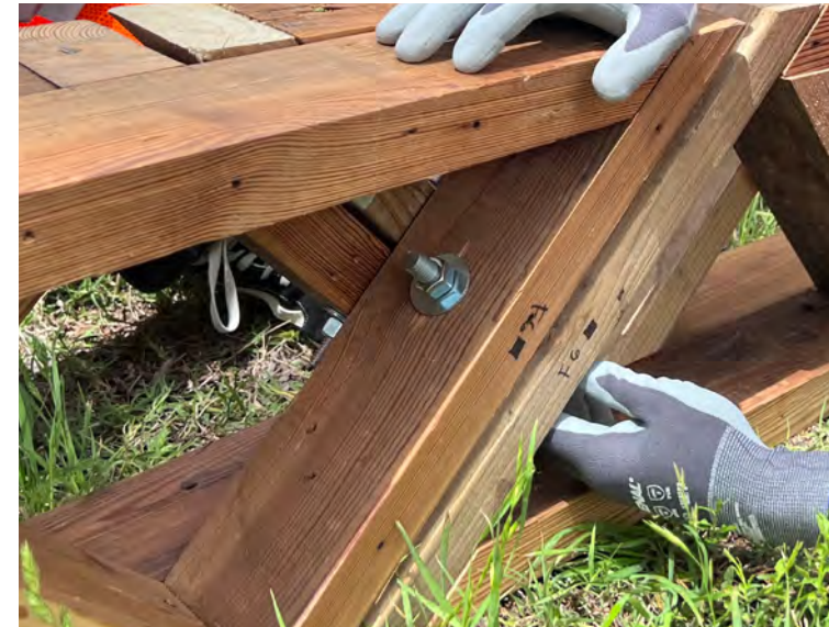
Figure 76 Connection bolt detail
