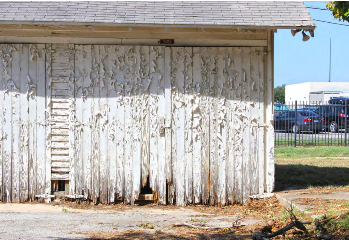
Figure 7 Garage door bottom deterioration due to rain exposure.
