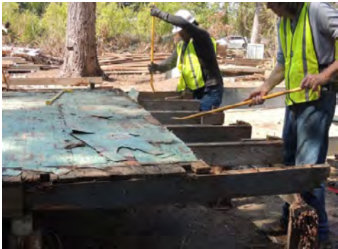
Figure 28 Deconstruction of a floor slab
