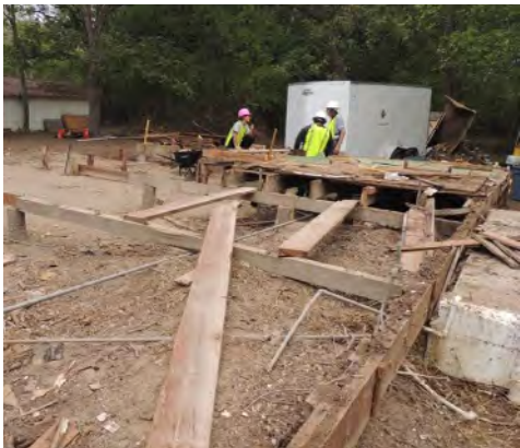
Figure 32 A pier and beam foundation
