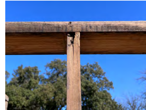
Figure 61 Defect in the connection of the framing stud
