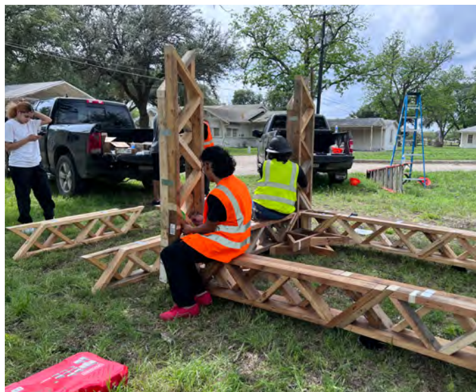
Figure 75 Half assembled prototype with truss blocks
