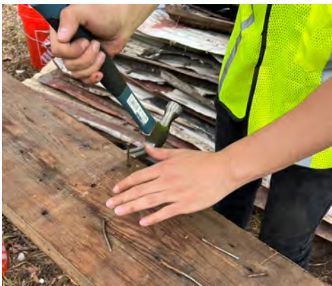
Figure 33 Denailing process
