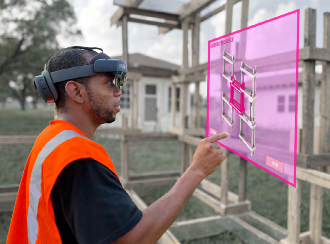
Figure 87 Illustration of the AR assembly instructions
